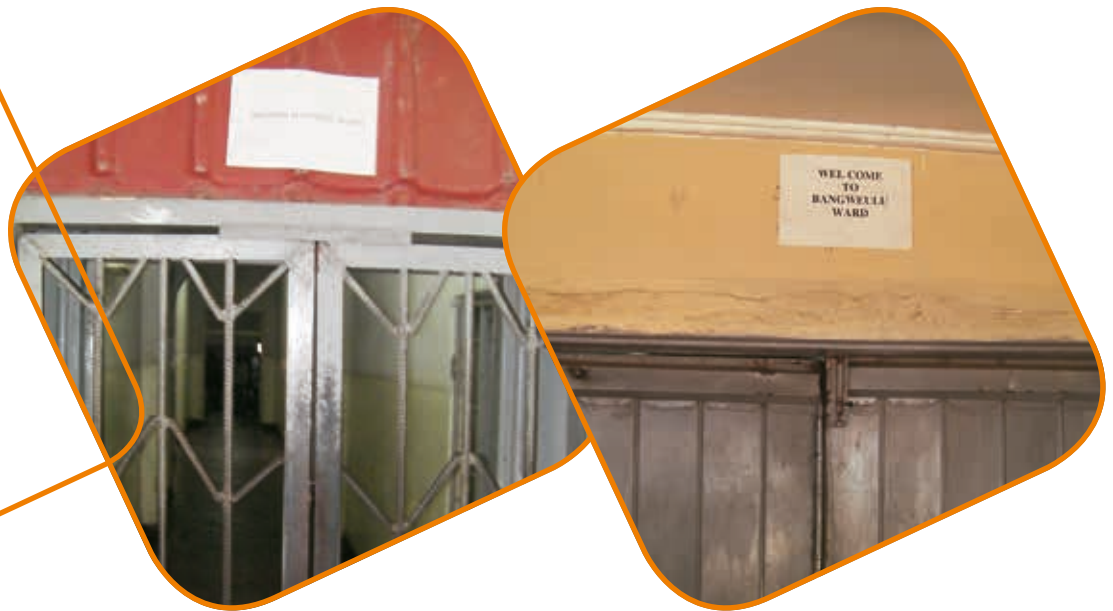
Photos: Entrance of Ndola male ward (left) and female ward (right), 24 October 2012. © MDAC.
