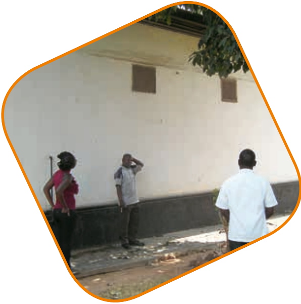
Photo: Staff expressed their regrets to monitors that the windows of the psychiatric ward at Ndola Hospital were built so high up, saying that they had had a limited understanding of mental health issues in the past, 24 October 2012. © MDAC.
